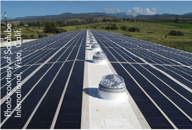
A combination of tubular daylighting devices and skylights provide natural daylight in the Kauai Island Utility Cooperative Port Allen Generating Facility in Eleele, Hawaii.
