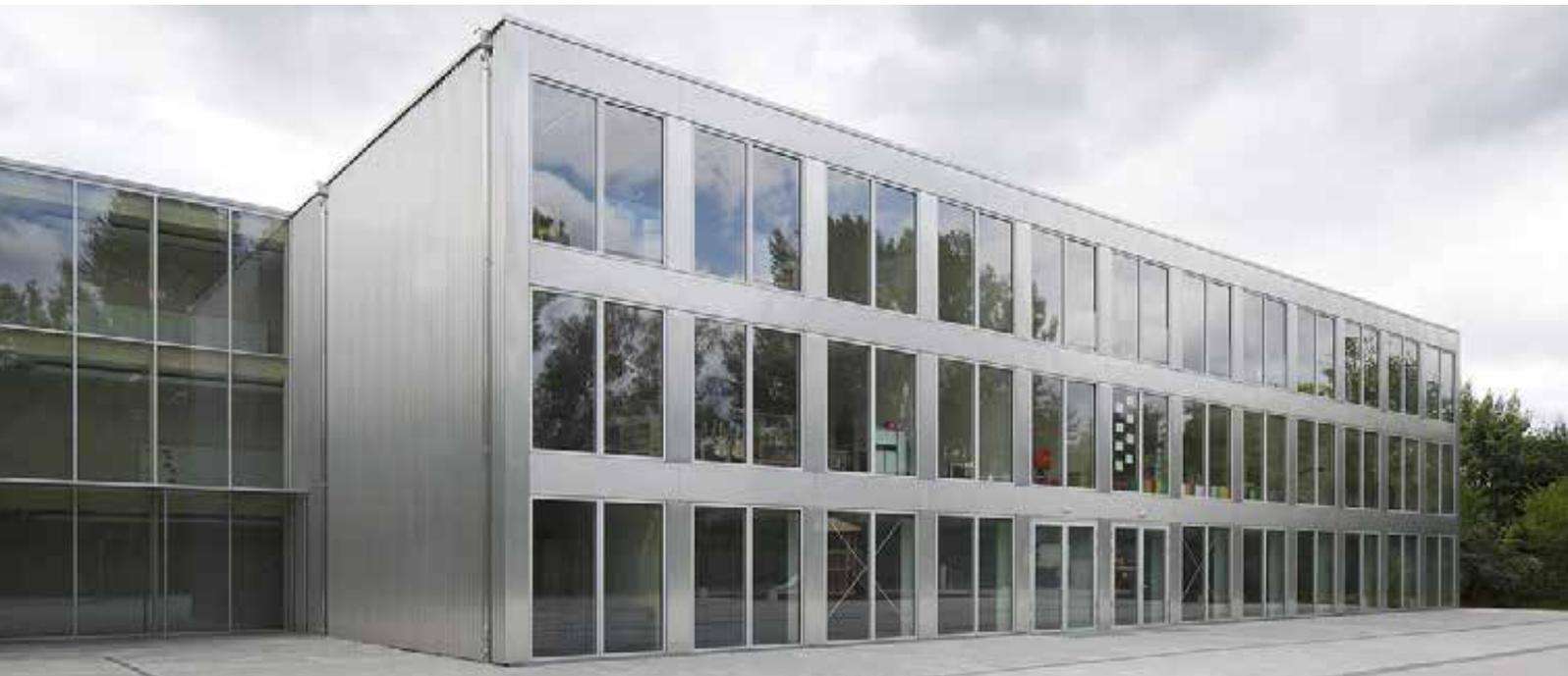
*Corrugated, perforated, and matte aluminum cladding make up much of the school’s exterior. But generous tripleglazed windows allow views to the surroundings and make the wood construction visible, even from the outside, so children can see and understand the building’s structure.*
