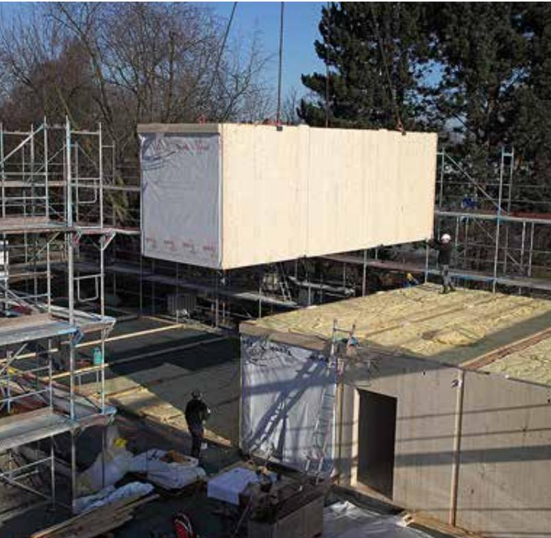
The modules were stacked on a slab and fastened to create a three-dimensional frame stiffened by the stairwell walls.
