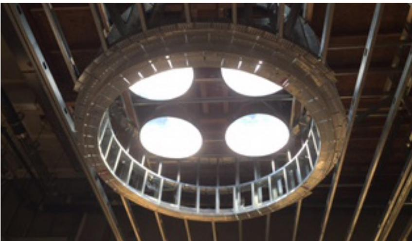
“Bringing in daylight to a two-story lobby was no small feat,” according to Angela Chiang, LEED AP, Project Designer at LPA, Inc. “We chose a unique configuration of four SkyVault units with Amplifiers installed as a group in one large nine-foot diameter lightwell.”
