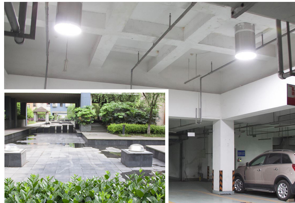
Underground Parking Structure
