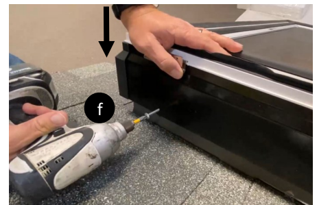
Insert snap spacer(s) between fastening hole and curb
